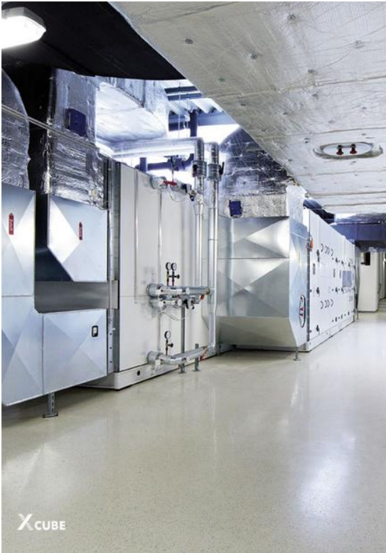
X-CUBE air handling unit
