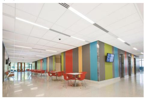
Inconspicuous integration of technical components: The TROX slot diffusers made of high-quality extruded aluminium sections blend in perfectly with the TECHZONE $^{\text{TM}}$  ceiling system.
