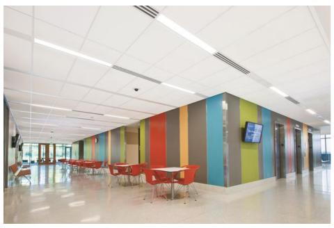
Inconspicuous integration of technical components: The TROX slot diffusers made of high-quality extruded aluminium sections blend in perfectly with the TECHZONE<sup>™</sup> ceiling system.
