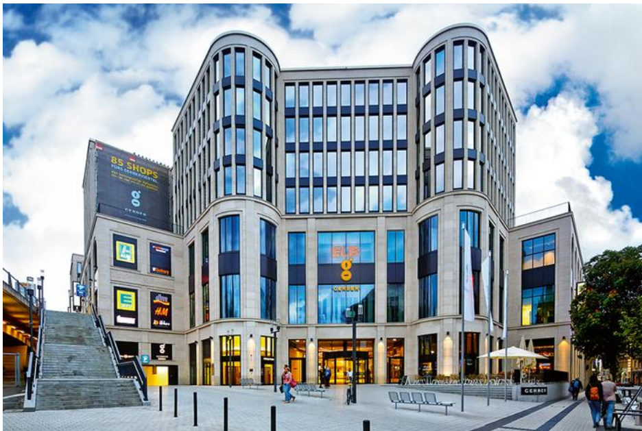
The GERBER shopping mall in Stuttgart is equipped with TROX products from air terminal devices to fire and smoke protection systems to air handling units
