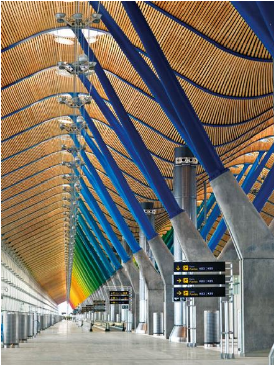
Madrid Barajas Example of combined displacement flow and mixed flow systems (jet nozzles)
