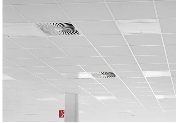
The volume flows of the TROX AIRNAMIC swirl diffusers are controlled with VAV terminal units and X-AIRCONTROL – on demand.
