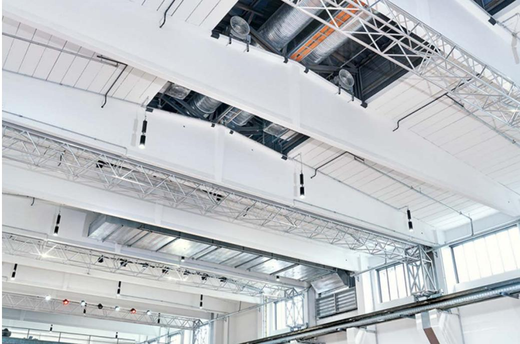
*Ten BVAXO smoke exhaust fans remove the smoke in the event of a fire.*
