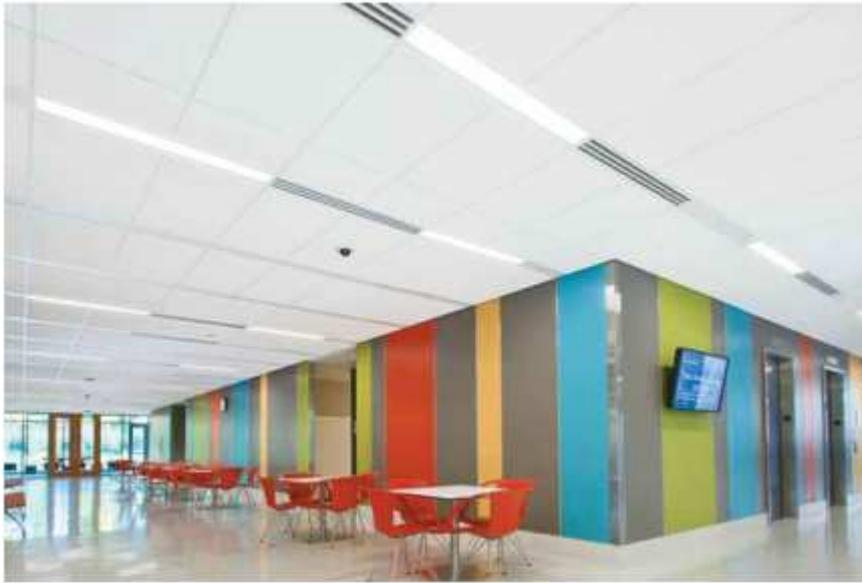
*Inconspicuous integration of technical components: The TROX slot diffusers made of high-quality extruded aluminium sections blend in perfectly with the TechZone ceiling system.*
