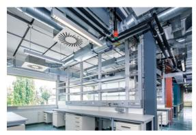
Ventilation and air conditioning in laboratories have to meet specific, extremely stringent safety requirements since their purpose is to protect the people working in these labs. TROX provides bespoke solutions that set new standards for research facilities and laboratories all over the world:
