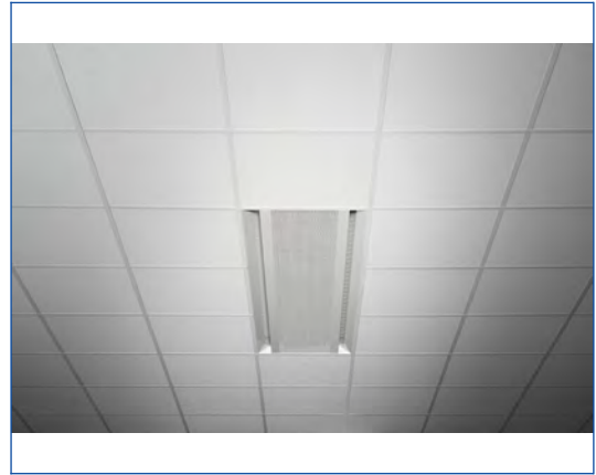
Installation into T-bar ceilings
