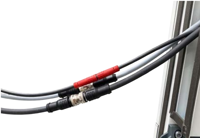
Fig. 41: Connection of the cables
