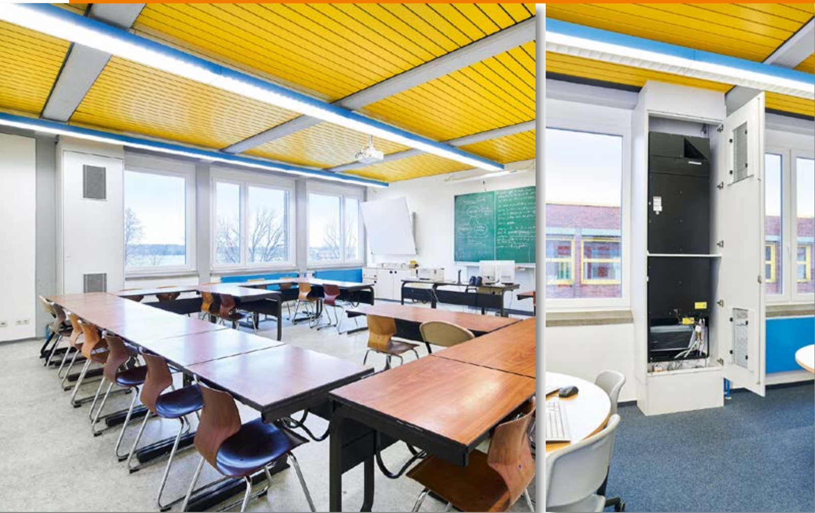
SCHOOLAIR-V vertical ventilation unit at the Paul-Spiegel-Berufskolleg vocational college in Warendorf, Germany.
