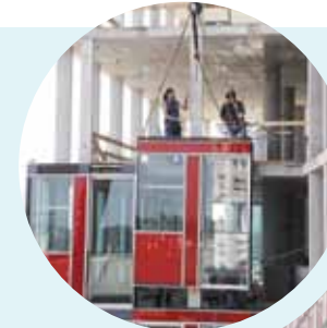
Example of an air-water system integrated in the façade: Capricorn office building in Duesseldorf, Germany.
