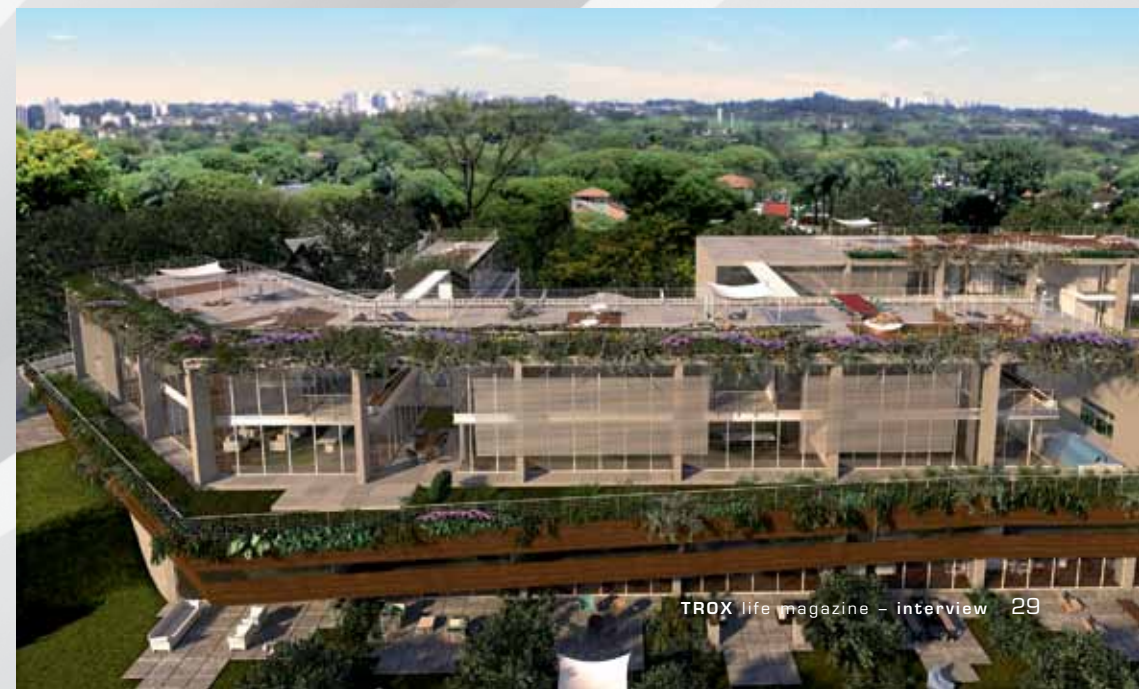
FGMF's Edifício Corujas project epitomises a triad philosophy of harmonious integration, quality of usage, and sustainability.
