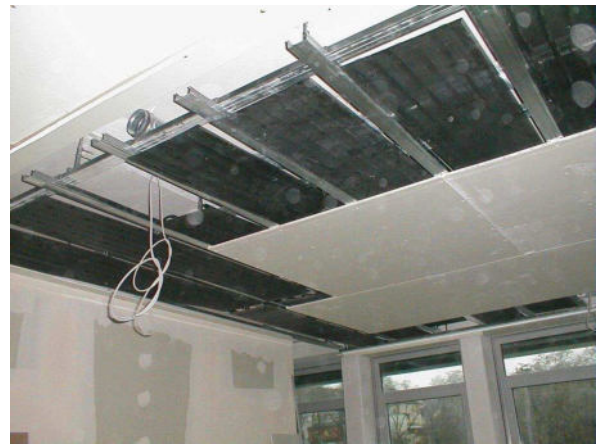
WK-D-GK with started plasterboard ceiling
