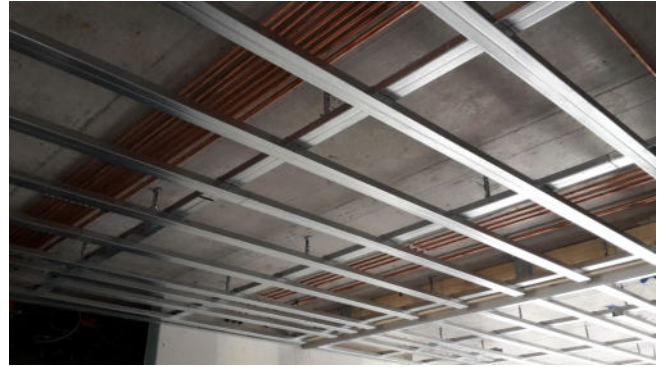
On-site support structure
